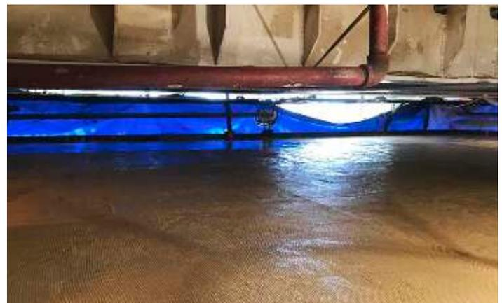
APPLICATION COMPLETED WITH FINAL COAT OF BELZONA 5831
