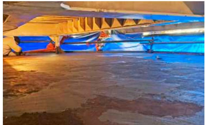
BELZONA 1161 APPLIED TO THE DAMAGED AREAS OF THE ROOF
